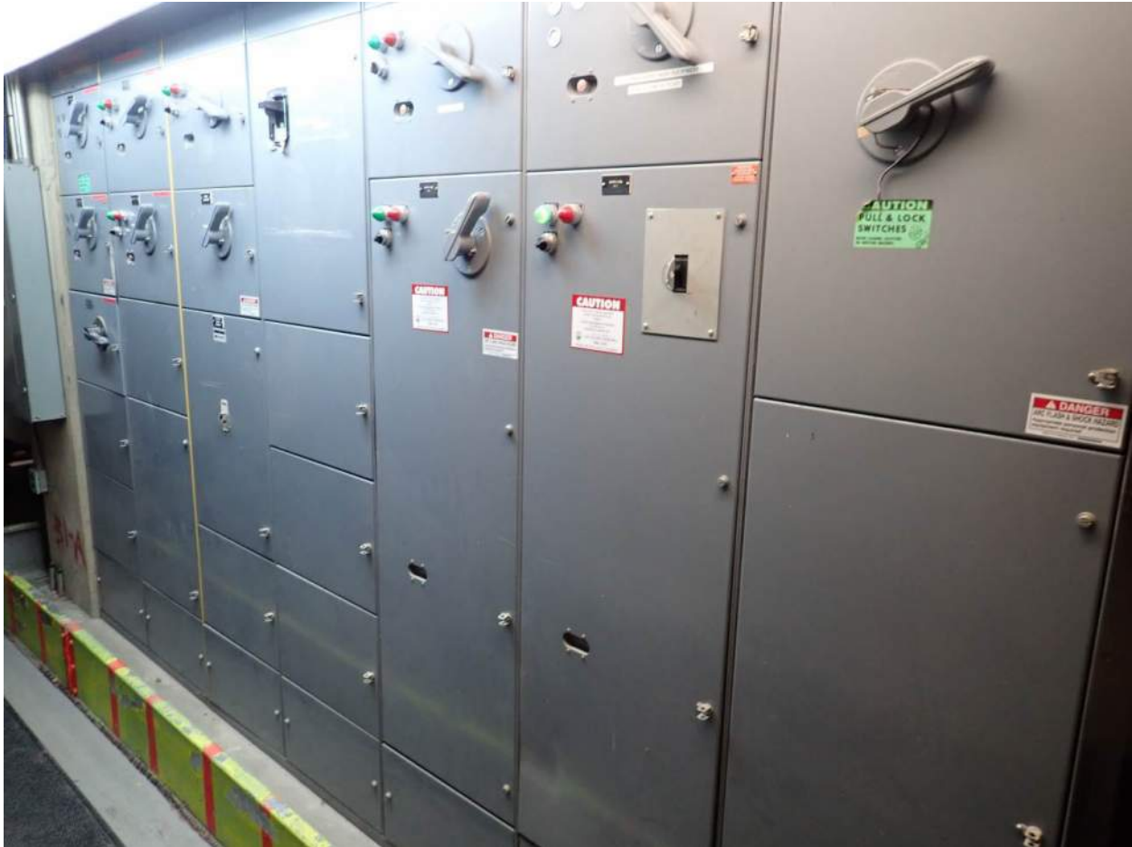
Photo 17 – Council Building MCC
